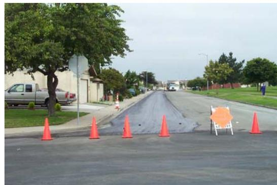
**Figure 18:** Road closures can be minimized by working in zones.
