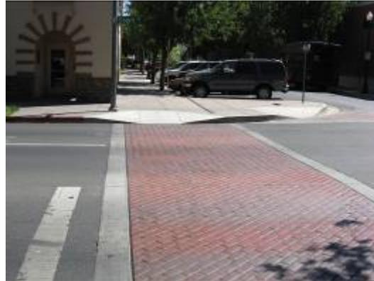
**Figure 11:** Stamped crosswalks are a trade-off between aesthetics and pavement maintenance costs.
