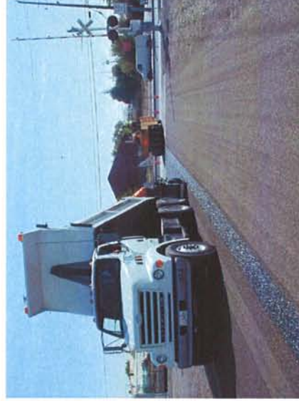
Driving in reverse prevents the truck from driving on the newly sprayed oil
