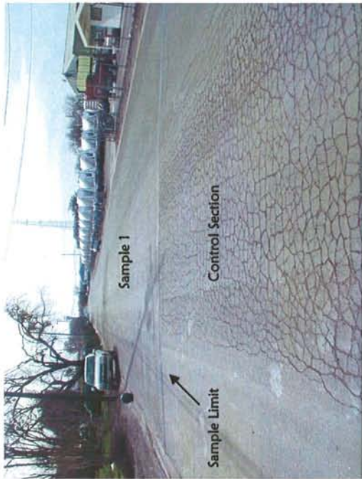
Control section is significantly deteriorated.
