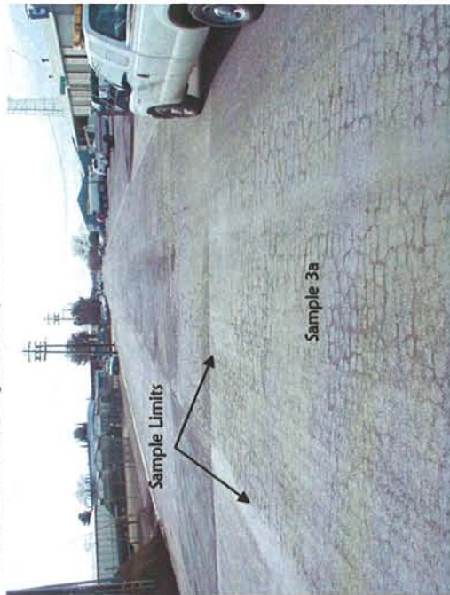
Control section is significantly deteriorated.
